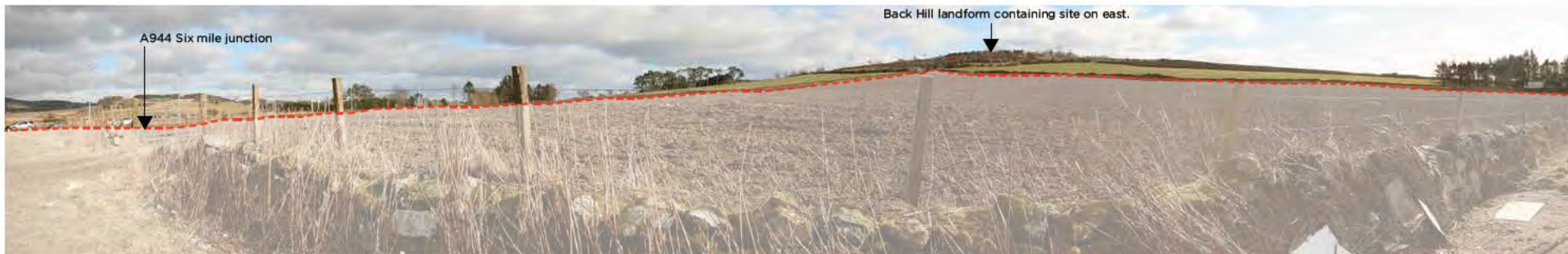
Panorama viewpoint 1: View from Westhill - Blacktop minor road at junction with B9119
