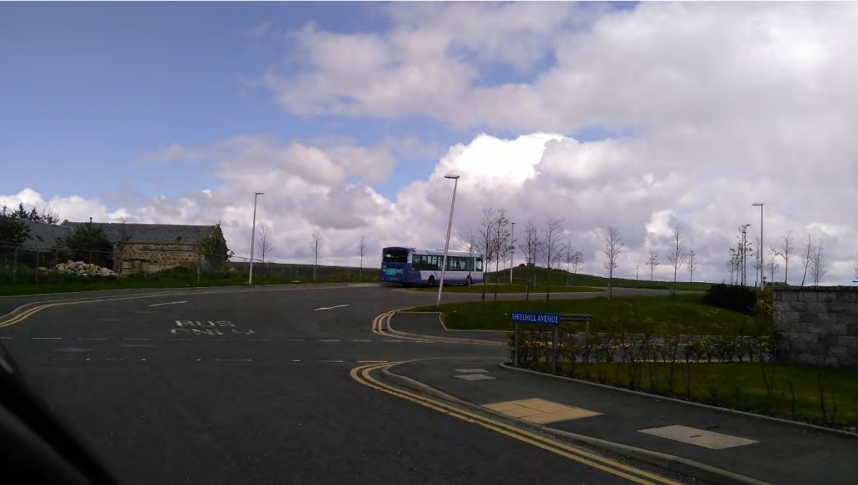
Figure 11 - completed bus terminus at Dubford
