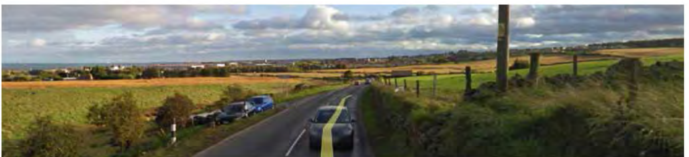
View of B999 looking south
