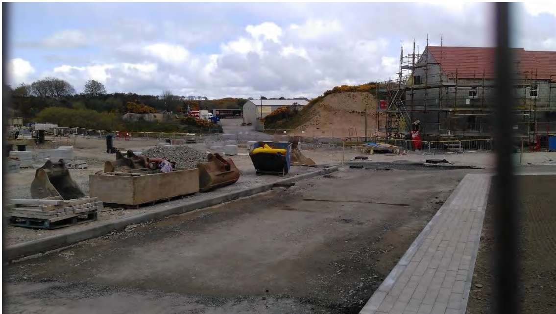
Figure 10 - development underway to south
