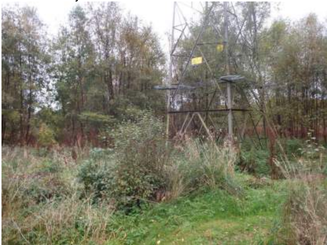
Photo 8: Electricity Pylon within central field
