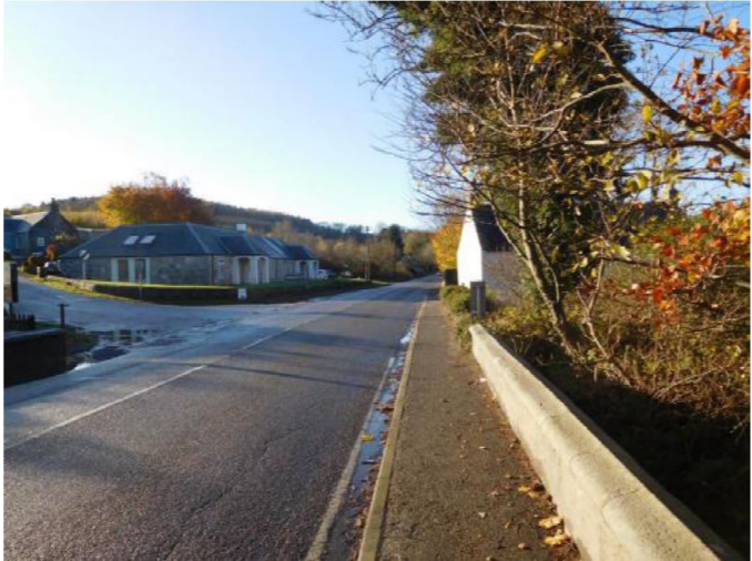
Figure 6b: B9077 at bridge crossing
