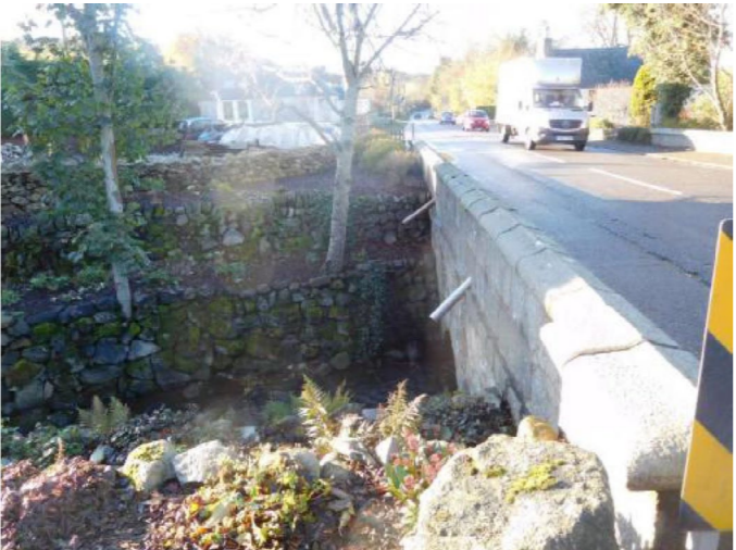
Figure 6a: B9077 bridge crossing
