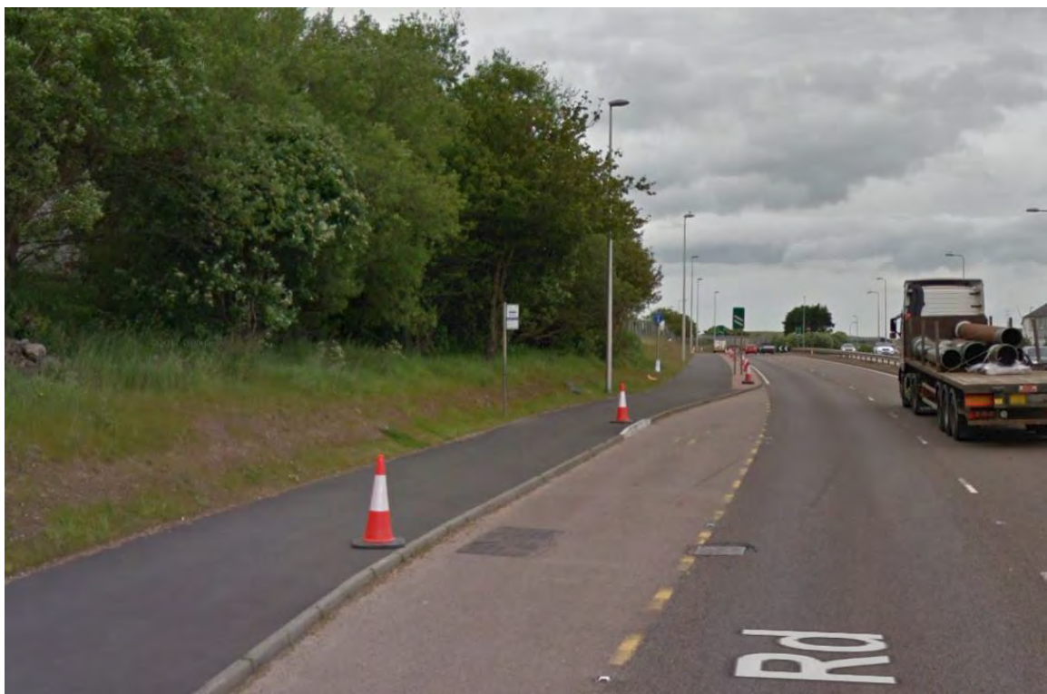
Figure 3.5 - A92 Cycleway/Footway Upgrade
