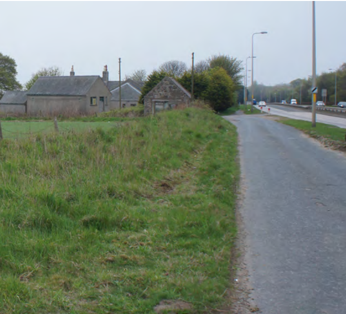
VIEW SOUTH TOWARDS ABERDEEN ENERGY PARK
