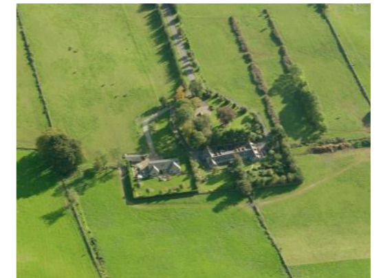
Aerial view showing existing properties at Craigbank....
