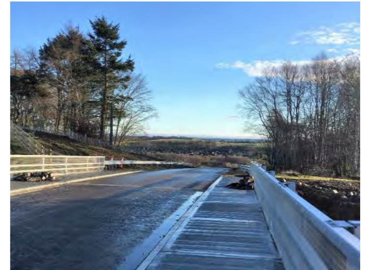
Photograph of the bridge over the AWPR (Aspirational Core Path)
