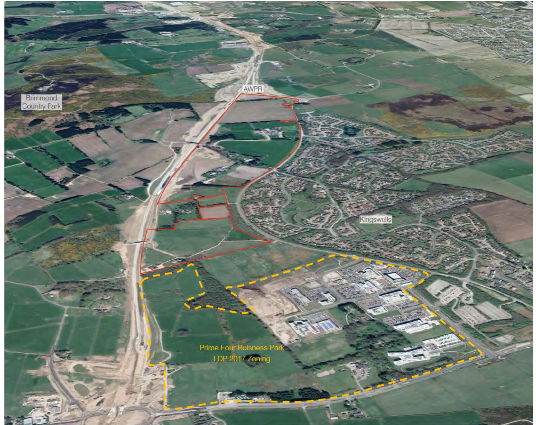
Aerial View of AWPR Works
