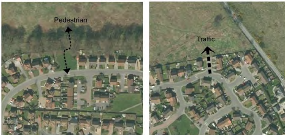
Figure 2 – Existing Wayleave/Access gaps
