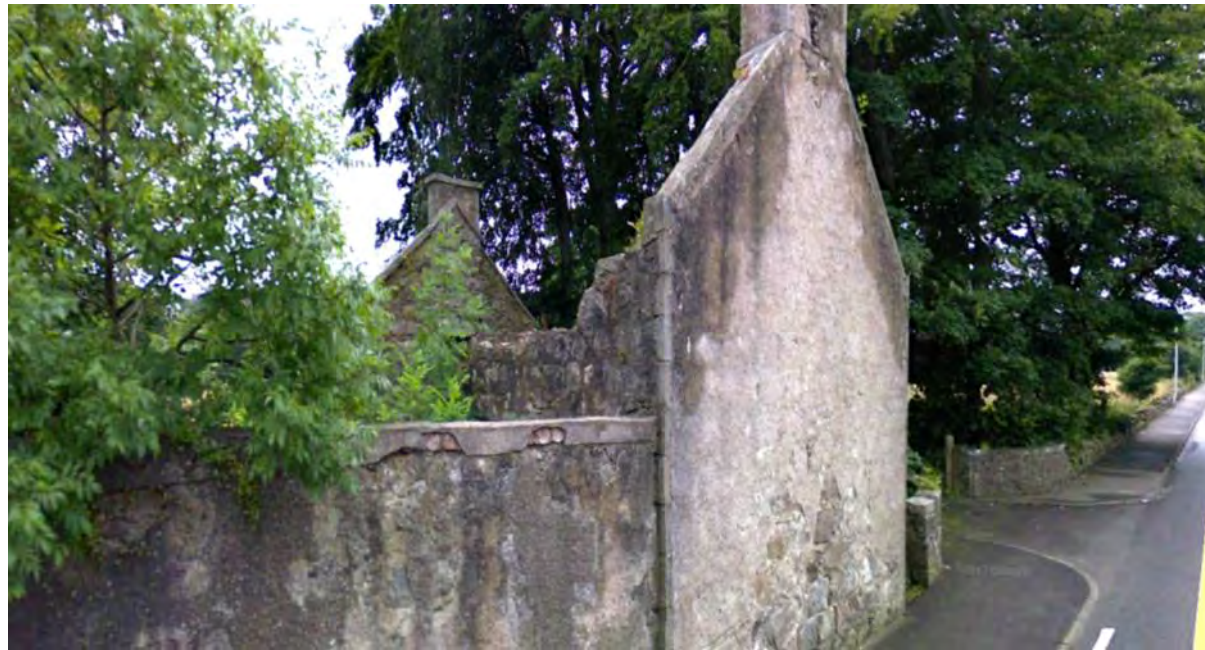
The redundant steading building to the North of the site - (Source: Google Maps)
