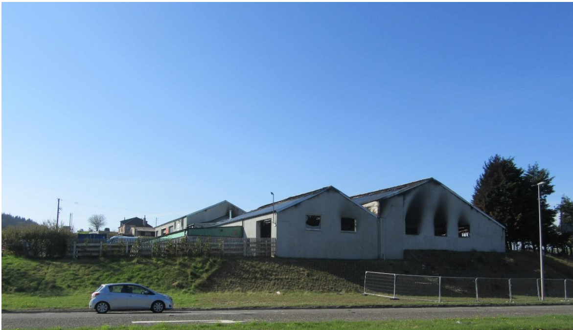
Figure 1: View to the site from the north showing fire damaged buildings.
