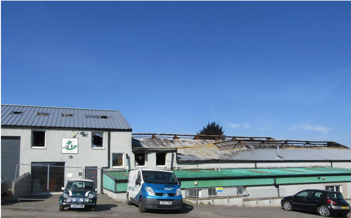
Figure 2: View of derelict buildings on site.
