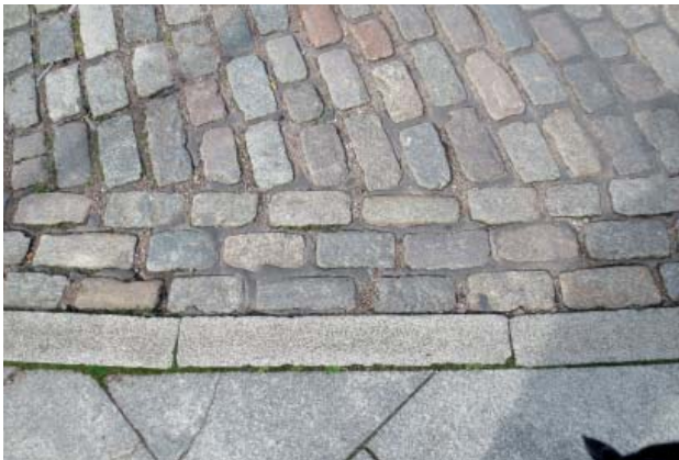
Relaid granite setts and paving, The Green
