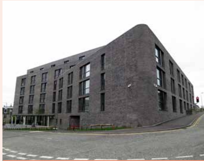
Grey brick used at 2 Powis Place student accommodation offers a successful contemporary contrast to the grey tones of Aberdeen
