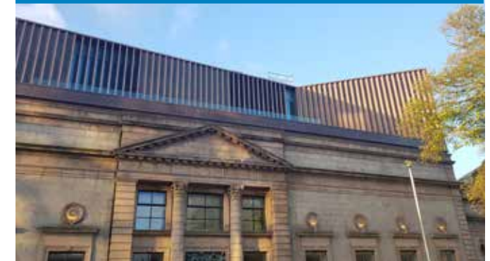
Aberdeen Art Gallery The contemporary roof extension to the Category 'A' listed Aberdeen Art Gallery has been designed as an honest, clearly modern addition to the original building and its granite façade below. The use of pink/brown copper cladding serves as a good match for the pink Corrennie granite used in the façade embellishments
