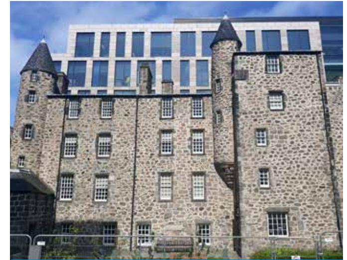
Marischal Square The use of new buff/brown granite cladding panels on the recent Marischal Square office development sympathetically reflects the colours seen in the walls of Provost Skene's House, one of Aberdeen's oldest buildings
