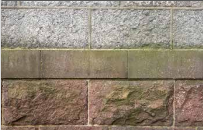
Aberdeen Art Gallery – the use of a rough-faced pink Corrennie base-course adds interest to the façade below the light grey Kemnay tooled blockwork.
