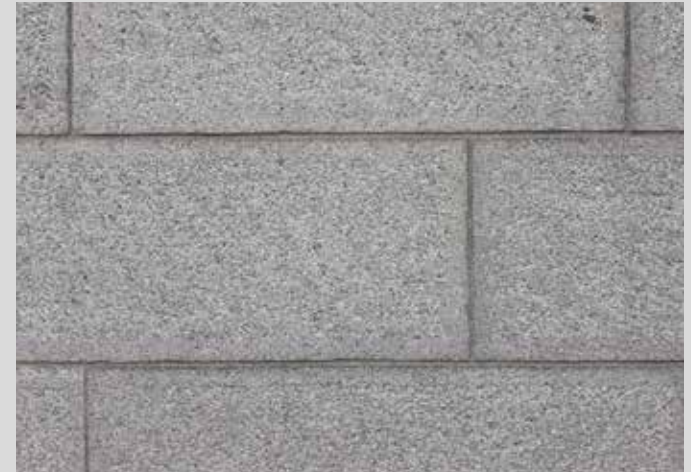
Ashlar blockwork – A standard light-grey ashlar-cut granite block. Ashlar blocks typically measure approximately 300mm-370mm in height and between 400mm and 800mm in length.
