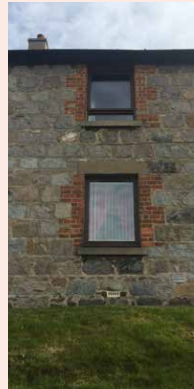
Granite wall with brick coping and window surround detailing – characteristic 'Seaton red'
