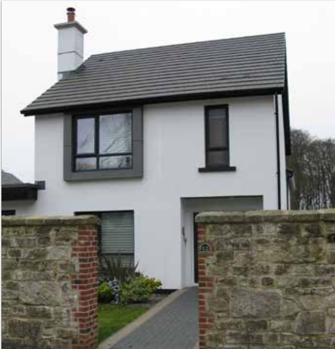
Smooth finish white render at Stoneywood – white render works well at 2-storey scale as is accessible and serviceable for maintenance
