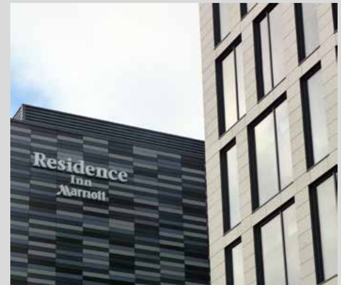
Imported granite cladding panels have been used successfully on new buildings in Aberdeen such as Marischal Square
