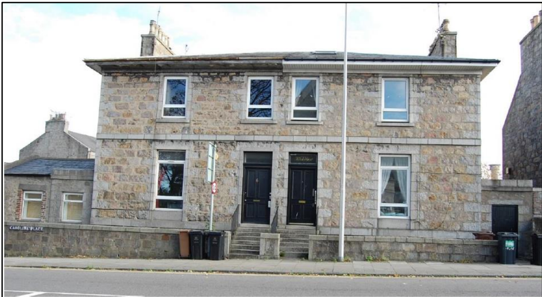
Photo: Façade of 6 Caroline Place
