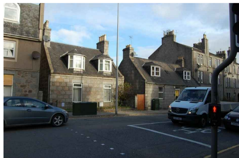
North side of Hutcheon Street, No. 166 to centre of photo
