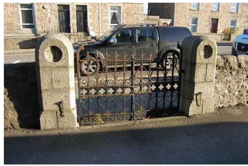
East entrance gates to The Fathers House (former Rosemount Parish Church); gates no longer open inwards due to change in ground level
