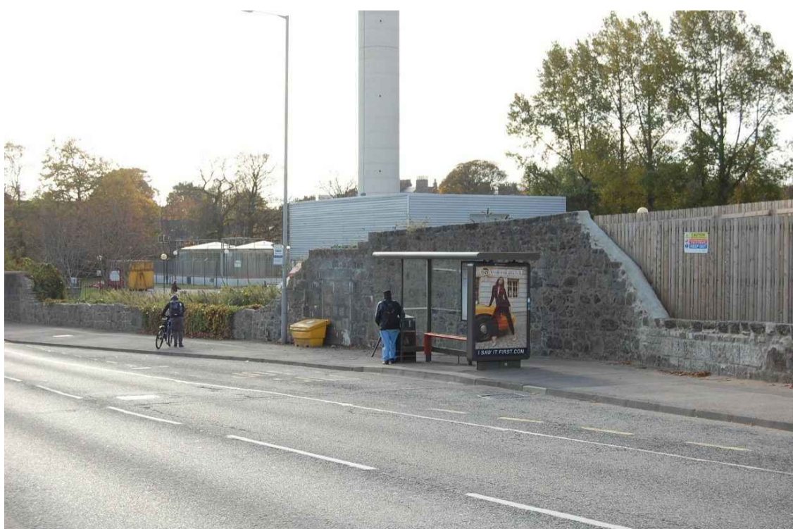
Boundary wall of Royal Cornhill Hospital adjacent to Berryden Road
