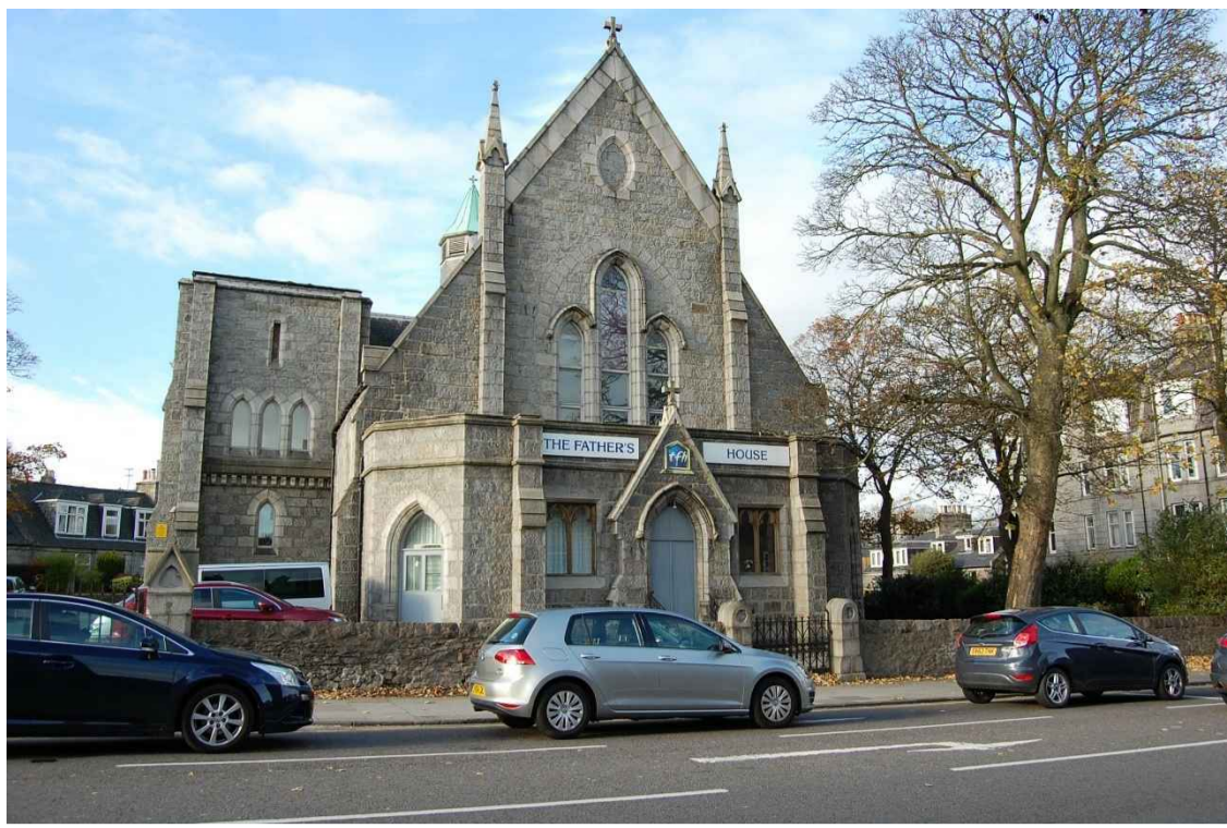
East side of The Fathers House (former Rosemount Parish Church)
