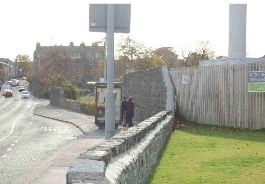
Boundary wall of Royal Cornhill Hospital adjacent to Berryden Road
