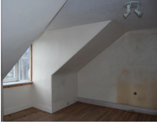
Figs.39, 40: Attic rooms, with water ingress, No. 2 Caroline Place
