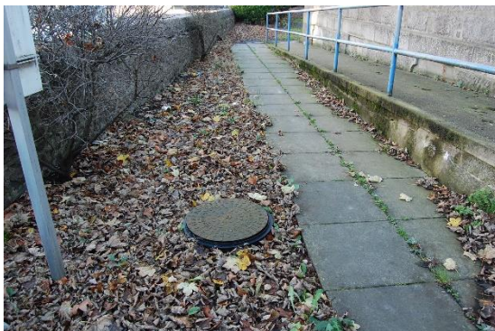
Fig.19: Ramp / wall at Westburn Road
