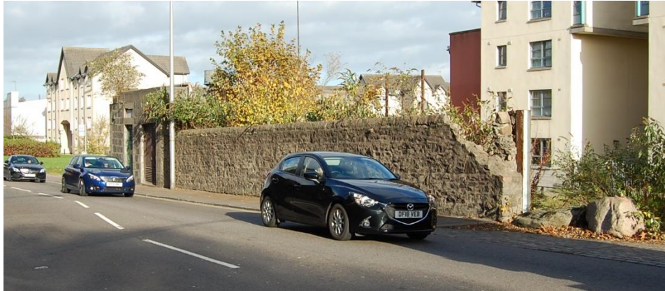
Fig.80: Berryden Road, remains of Industrial Building
