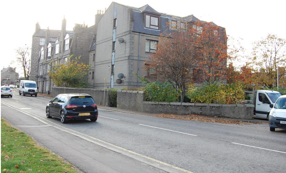
Fig.73: Berryden Road, South west: modern rendered wall to recent flatted development
