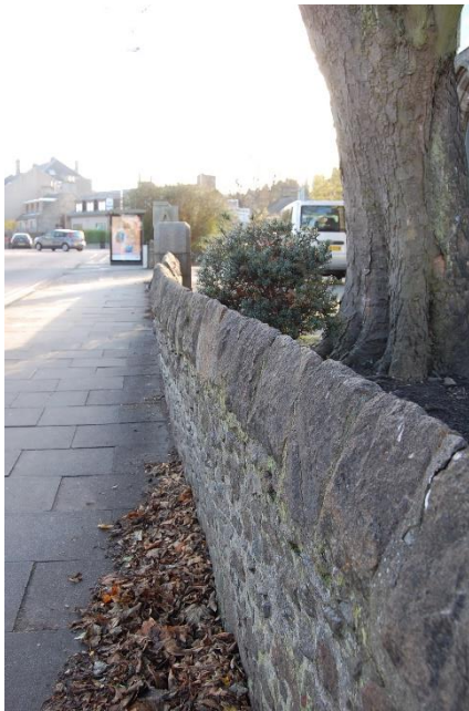
^Fig. 21: cement pointing, missing areas and cracking
