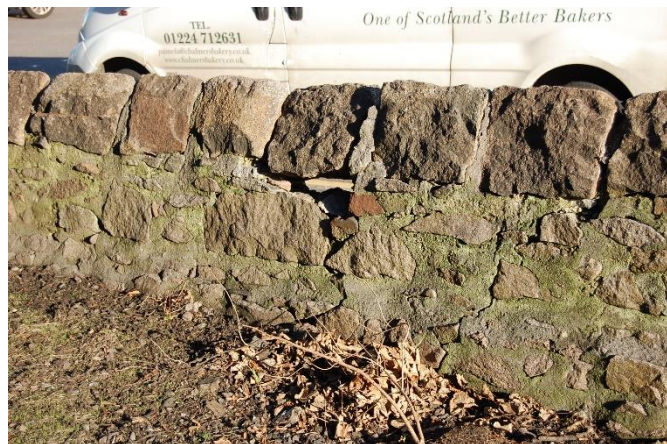
^Fig. 21: cement pointing, missing areas and cracking
