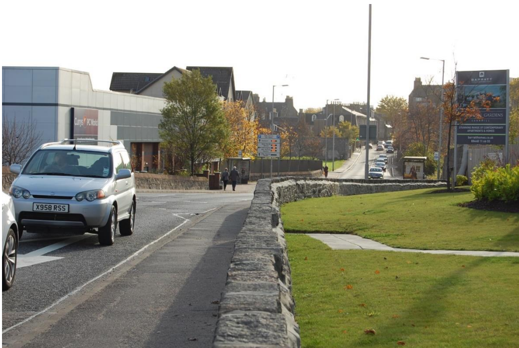
Fig.78: Berryden Road, former Asylum boundary walls to new housing development to west, recently reduced in height and capped.
