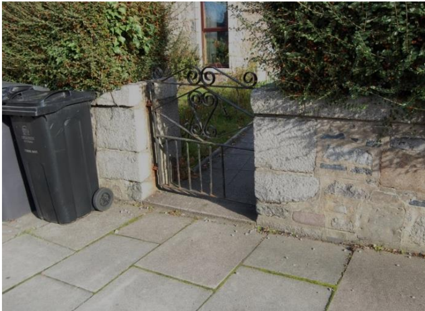
Fig. 24: Front gate and boundary wall, No. 1 Caroline Place.
