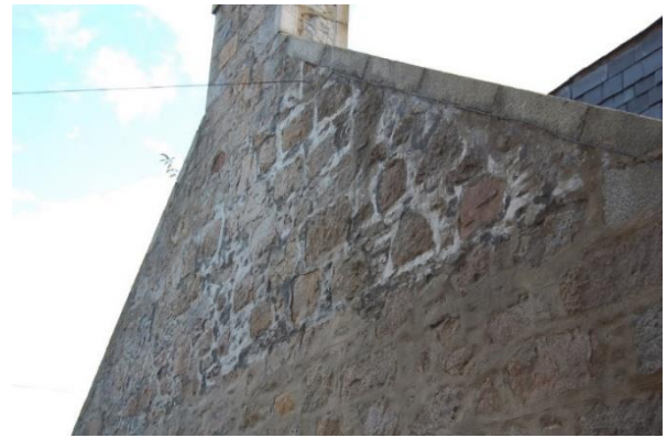
^Fig. 41: cement pointing to gables
