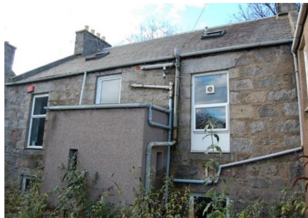
<Fig. 33: North extension block No. 2 Caroline Place
