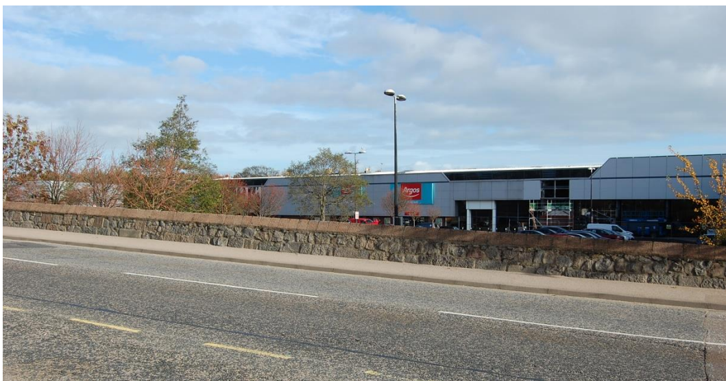
Fig.81: Berryden Road, boundary wall to Retail Park
