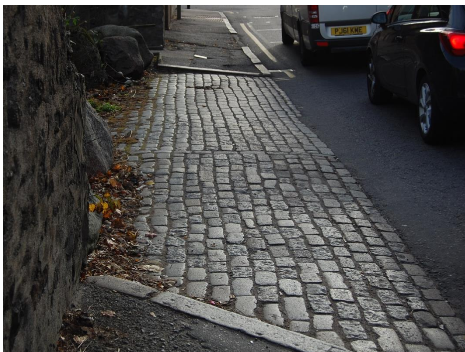
Fig.83: Berryden Road, granite setts and kerbstones to former mill entrance
