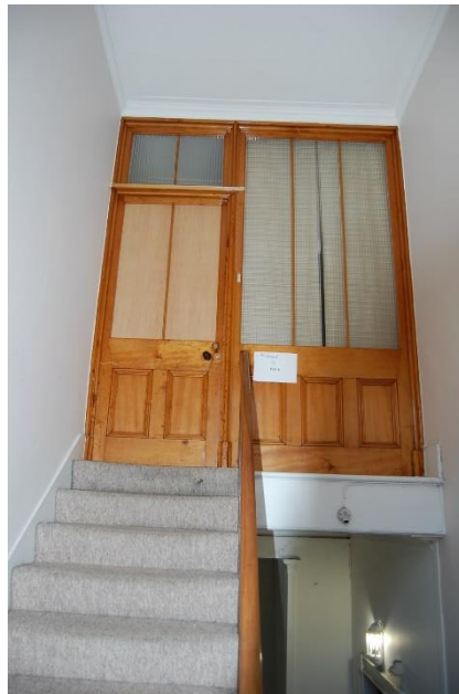
<<Fig. 56, 57: No. 6 main stair, ground and upper floor levels
