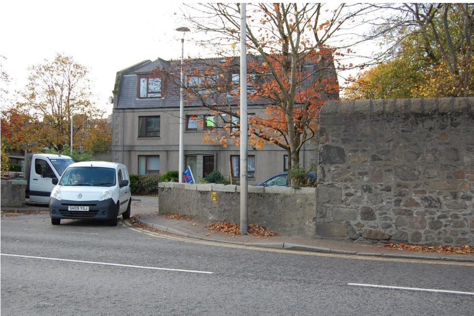
Fig.74: Berryden Road, southern edge of orchard wall to right.
