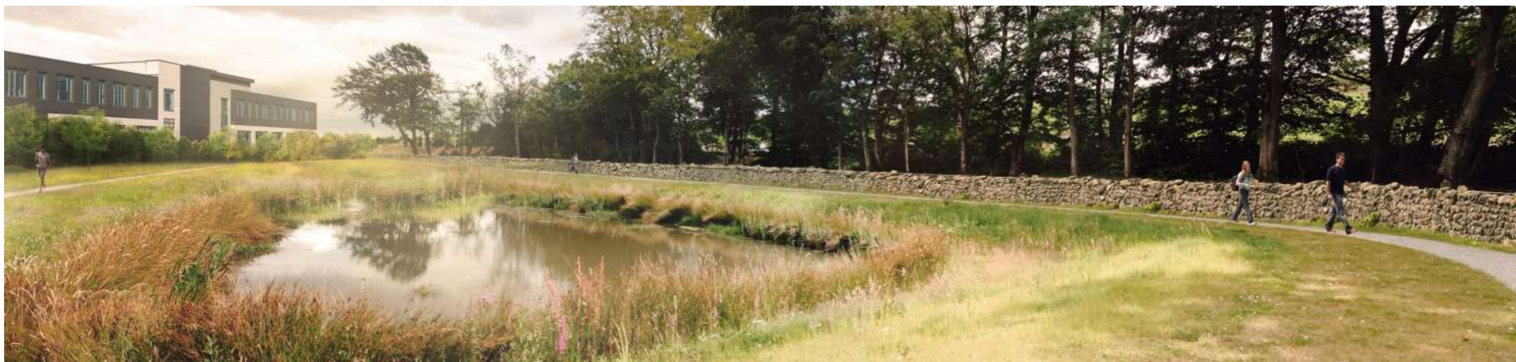
fig 51. indicative image of northern SUDS basin
