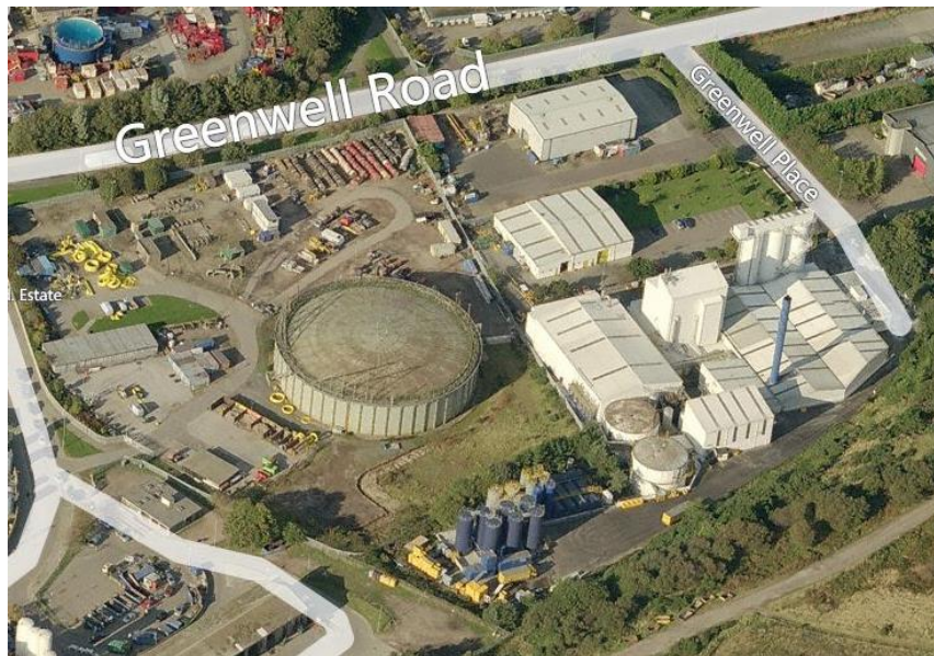
Aerial view of the Aberdeen Gas Holder Site
