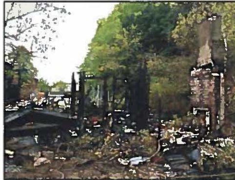
Photo 6: Fire damage to buildings
