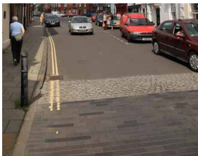
Change in carriageway material at pedestrian crossing
