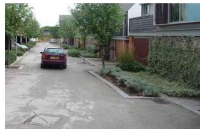
Shared surface and use of planting to reduce carriageway
