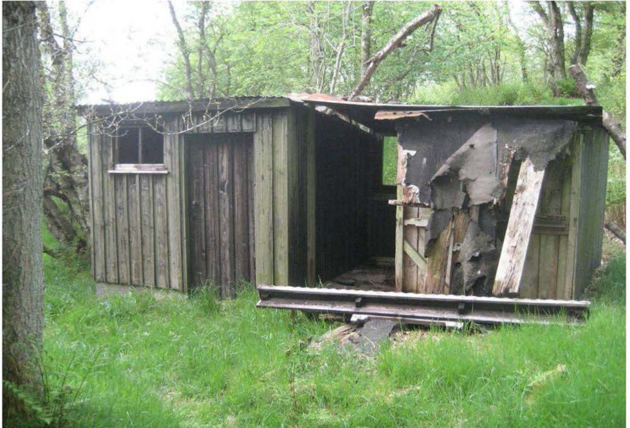
Figure 5 – Shed on Site
