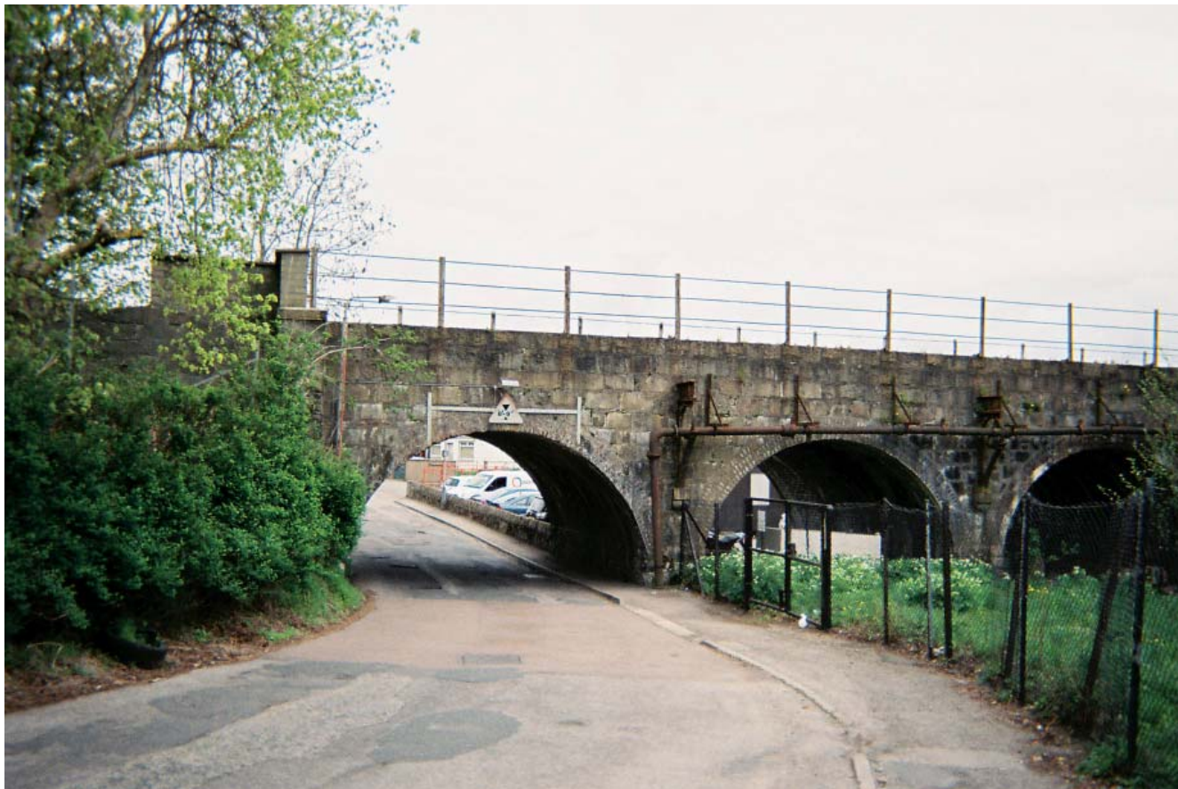
Old railway Bridge
