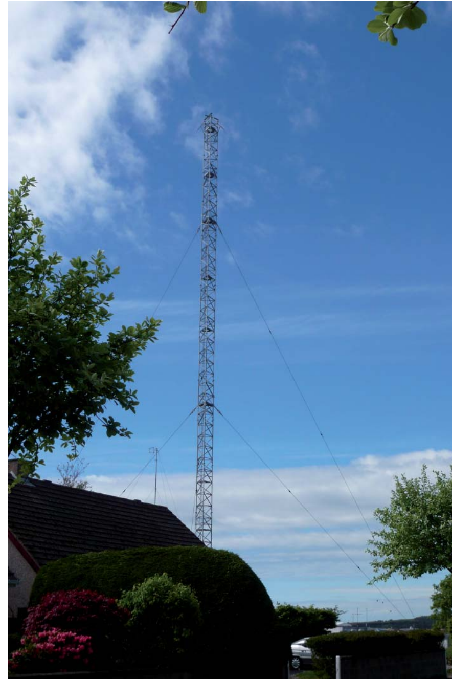
Redmoss Transmitter Houses 2
