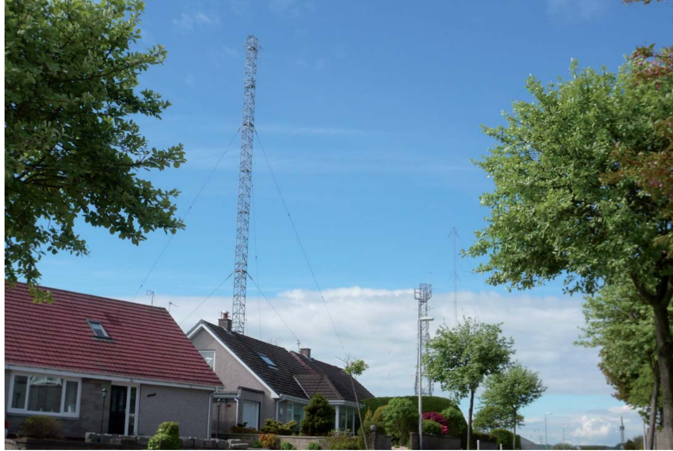
Redmoss Transmitter Houses
