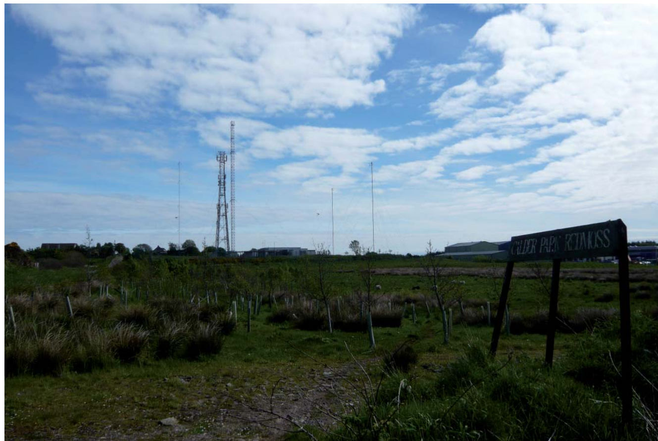
Redmoss Transmitter Clader Park School
