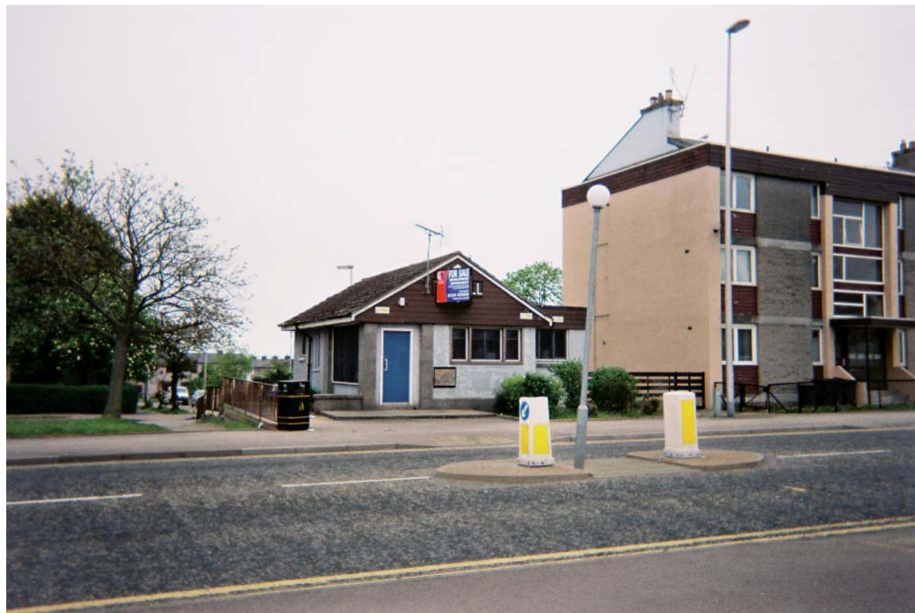
Former Police Box needs new use
