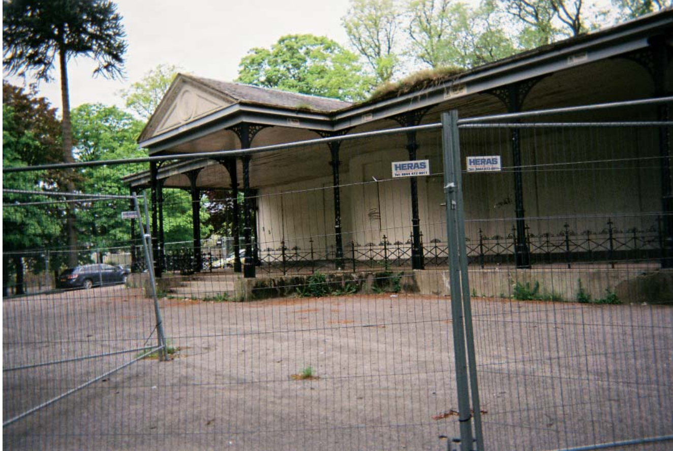
Derelict State of Westburn Villa
