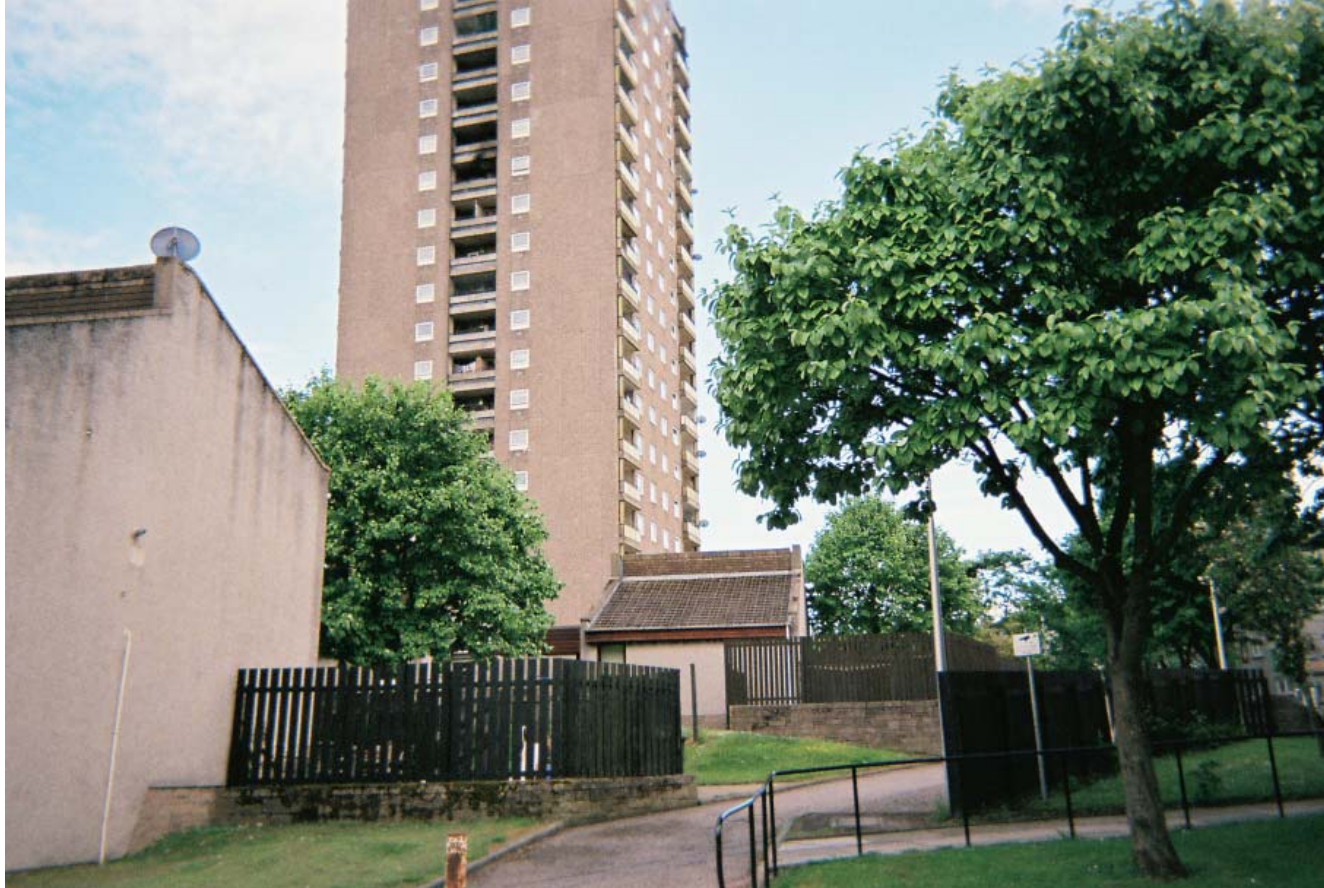
Ugly tower blocks
