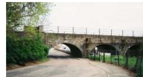
Old Railway Bridge
