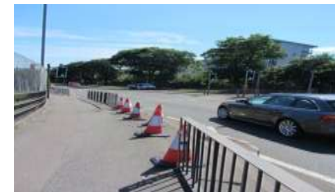
Pavements unsafe for pedestrians
