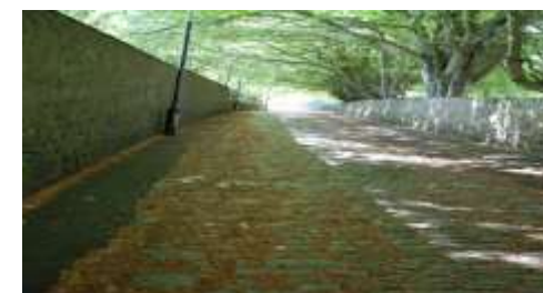
Poorly maintained cycle route unsuitable for cyclists
