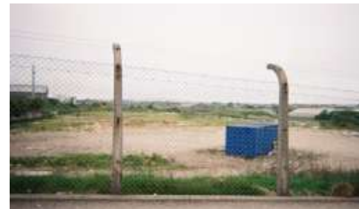
Large, long term derelict site at Granitehill
