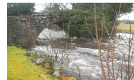
The Shoddy Pack-Horse Bridge over the Culter Burn
