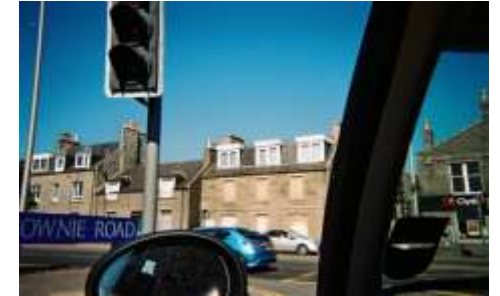
Empty, boarded up buildings
