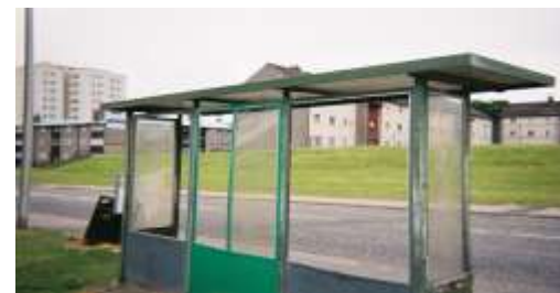
Bus shelter needs replacing
