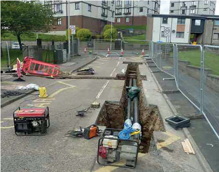
Pipe work for Torry Heat Network
