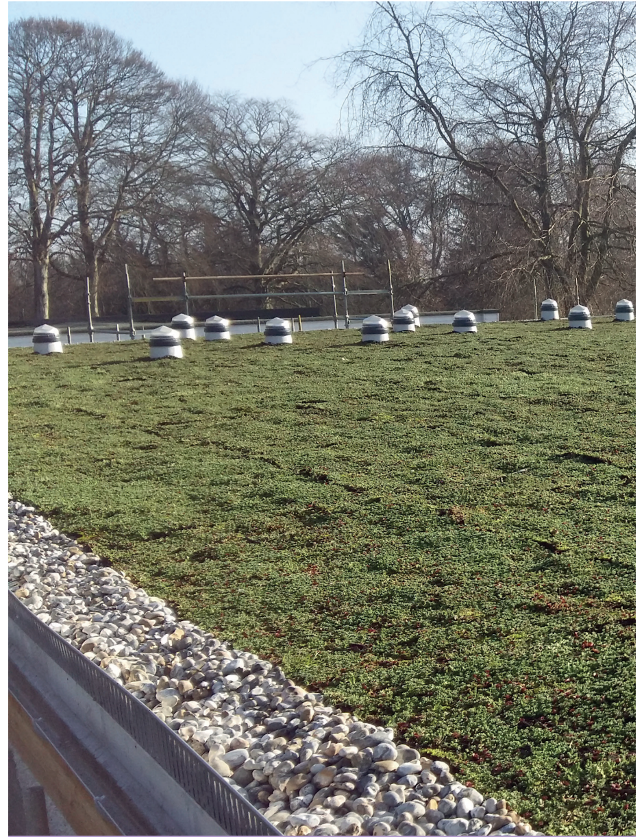
Green roof – Pets' Corner building, Hazlehead Park
