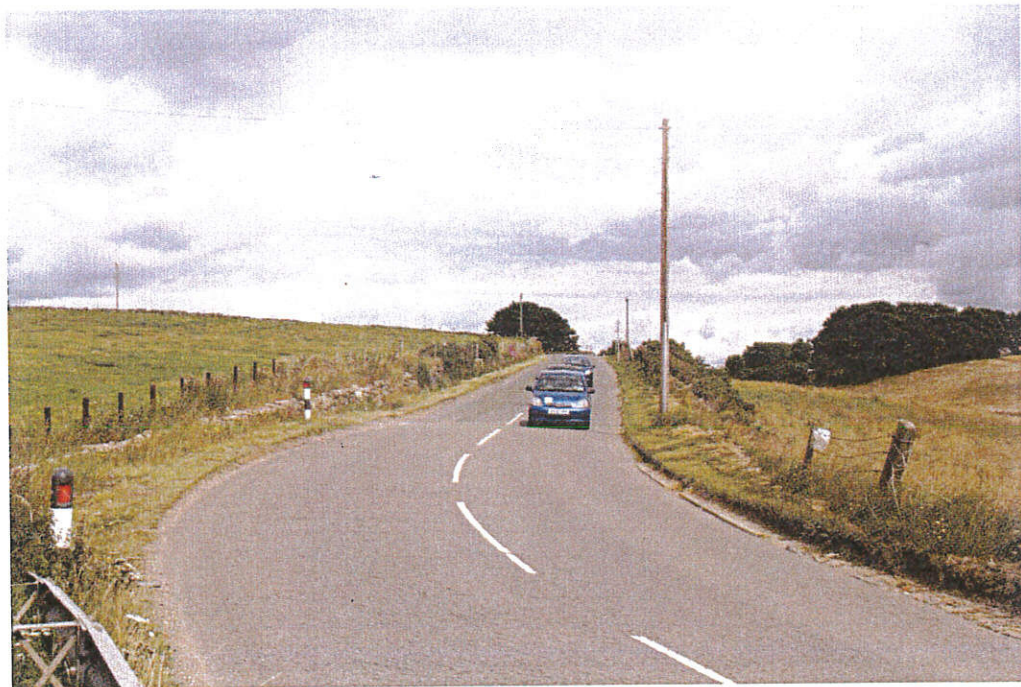
B999 looking north east towards development site
