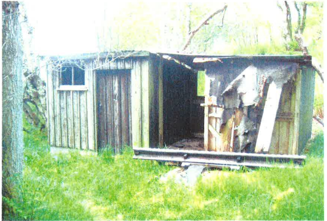
Figure 5 – Shed on Site
