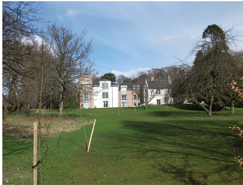
Retirement flats, Airyhall Road
