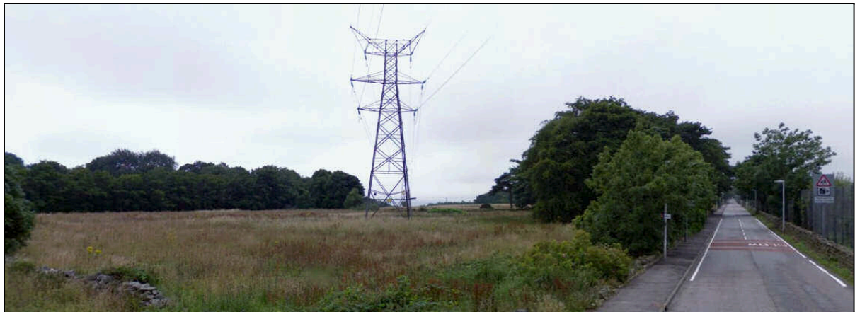
Fig 2 – the site is dominated by a line of pylons, but peripheral tree planting is of value.
