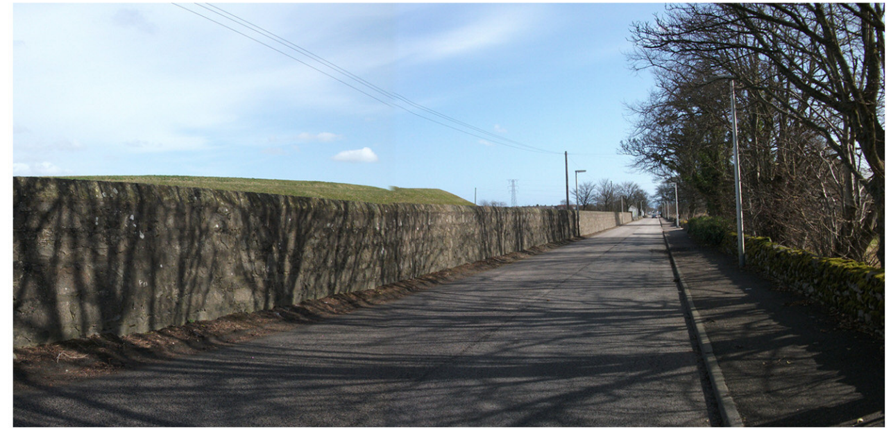
Covered reservoir from Craigton Road
