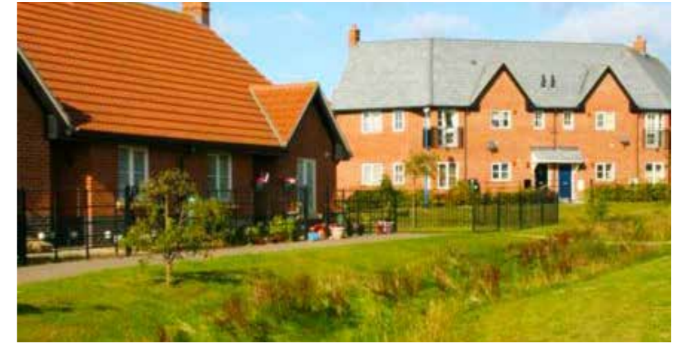
Integrated linear SuDS (Lamb Drove, Cambourne, Cambridgeshire)
