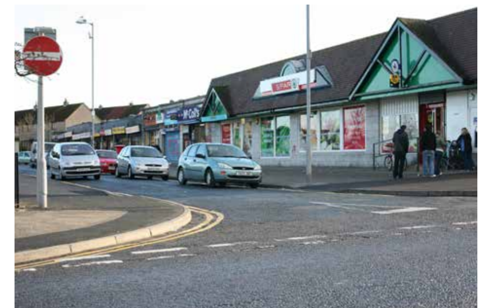
Fig. 34: Northfield Neighbourhood Centre.
