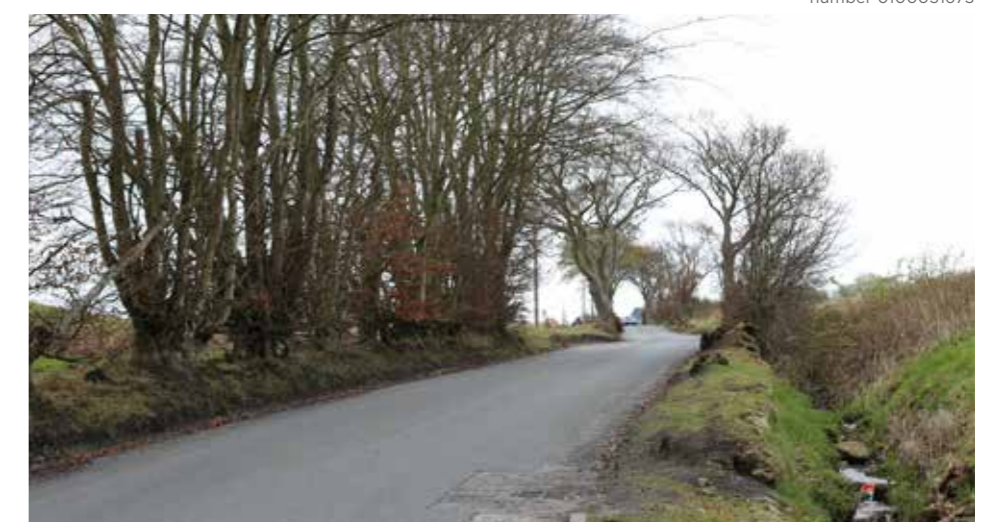
Fig. 18: Existing drainage ditches across the site.
