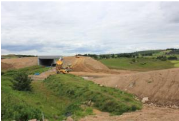
Construction of the Aberdeen Western Peripheral Route
