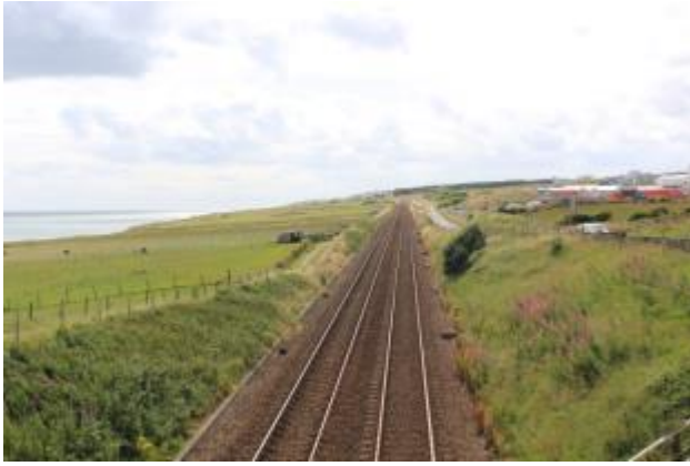
East Coast Mainline Railway and gently sloping fields
