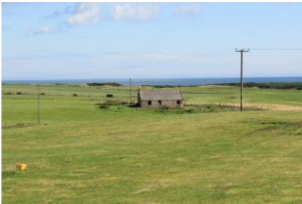
Derelict farm building
