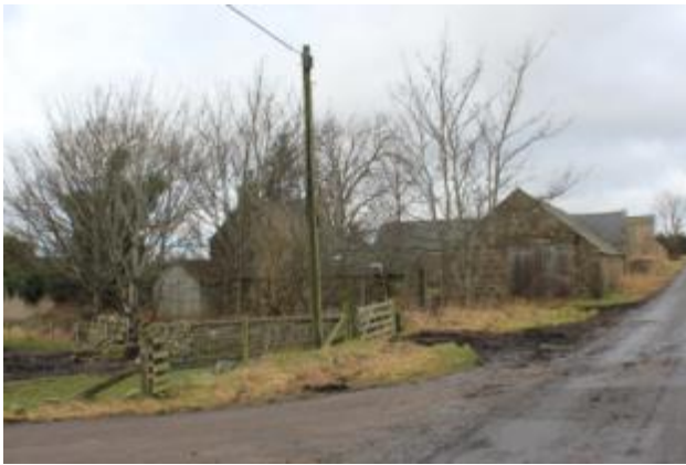
Derelict farm buildings
