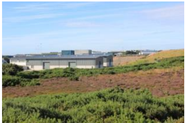
Nearby Tullos Industrial Estate
