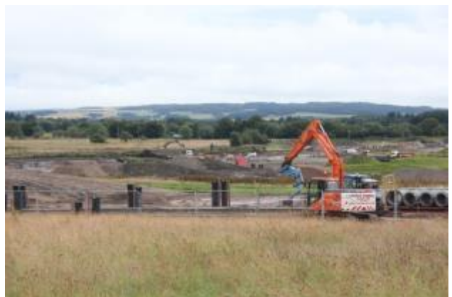
Recent construction activity of residential development
