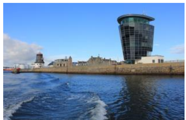
Marine Operations Centre building at harbour entrance
