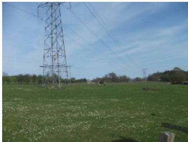
Pylons can appear visually intrusive
