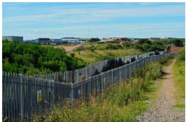
Fenced pipeline and industrial units beyond to the south
