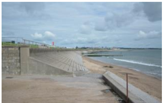
Concrete revetments and timber groins along the beach
