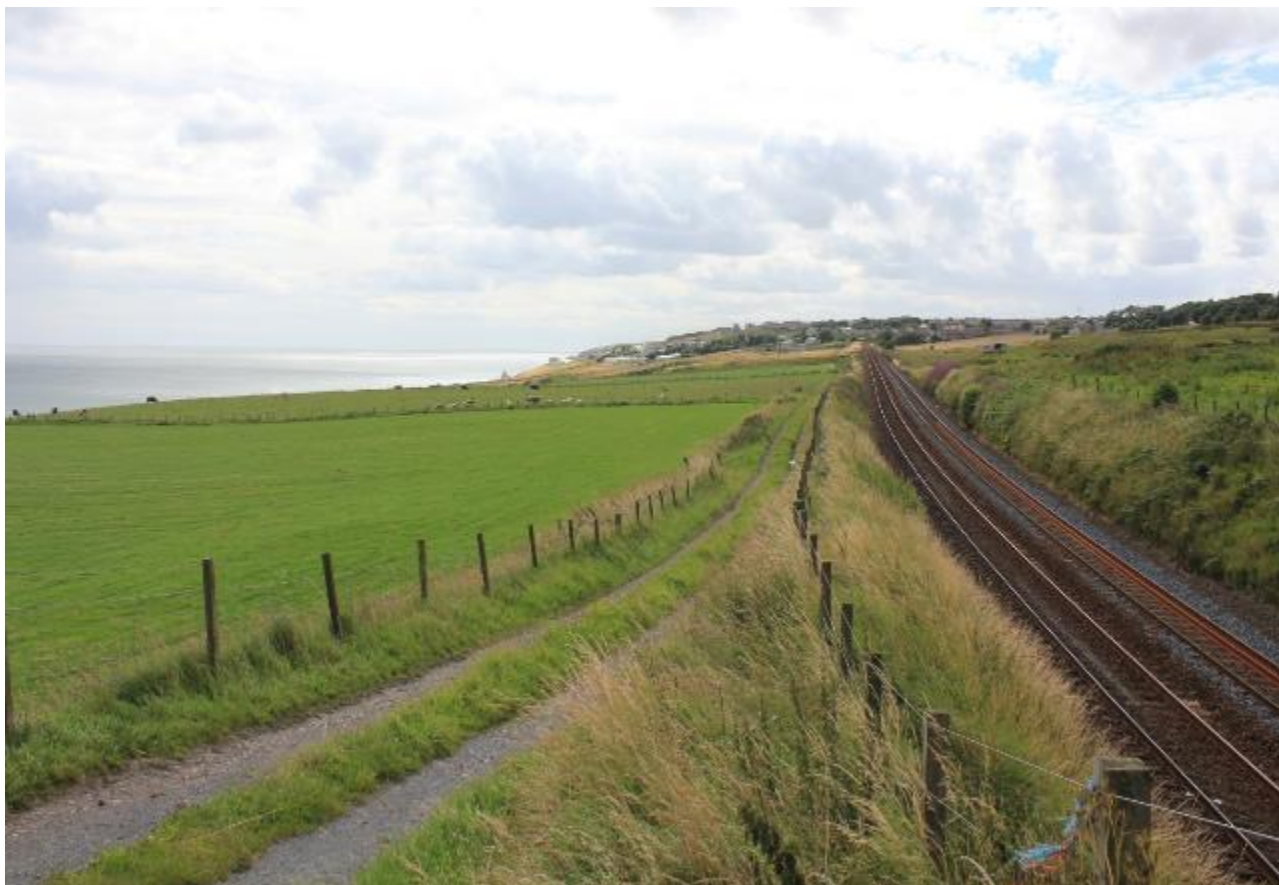
Looking south along the railway towards Cove
