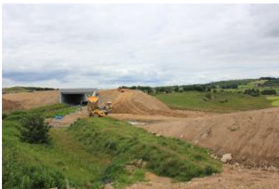
Aberdeen Western Peripheral Route construction
