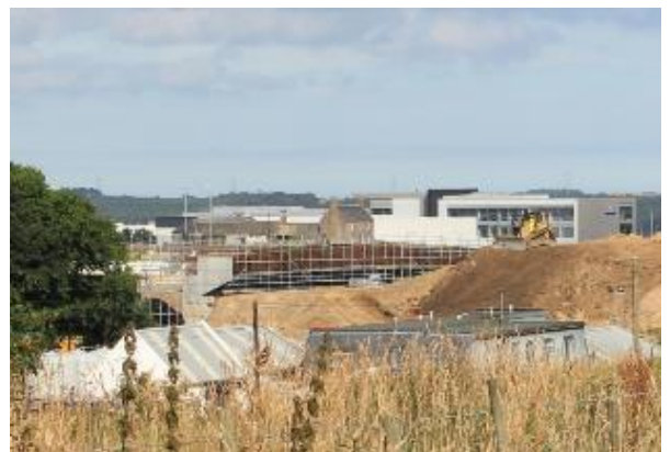
AWPR and business park construction along the A96
