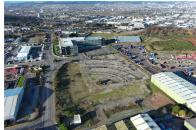
Vacant Business & Employment allocated land at the centre of Altens Industrial Estate – suitable for a mix of industrial typologies to support growing energy transition businesses.
