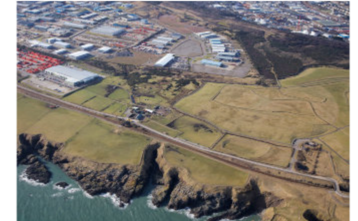
Brownfield land within Altens (Peterseat Drive) presents opportunity to integrate existing industrial sites and further expand the Campus
