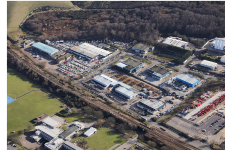
East Tullos Industrial Estate
