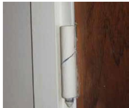
Figure 5 Rising Butt Hinge
