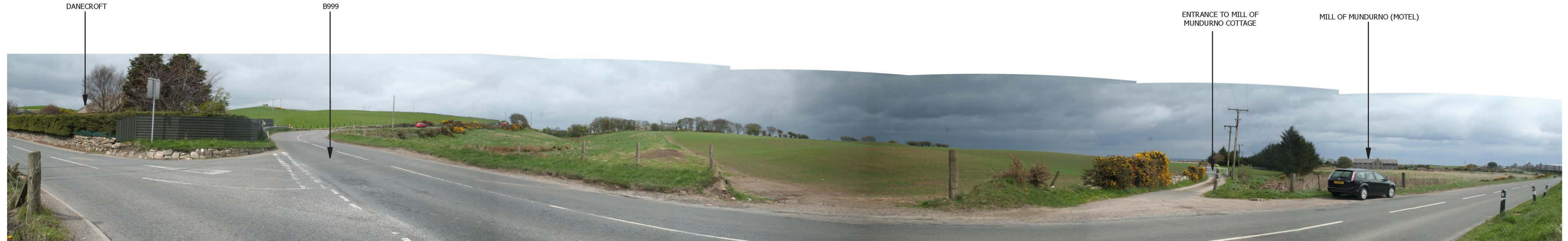
SITE CONTEXT PHOTOGRAPH 1: VIEW TAKEN FROM B999 LOOKING NORTHWARDS
