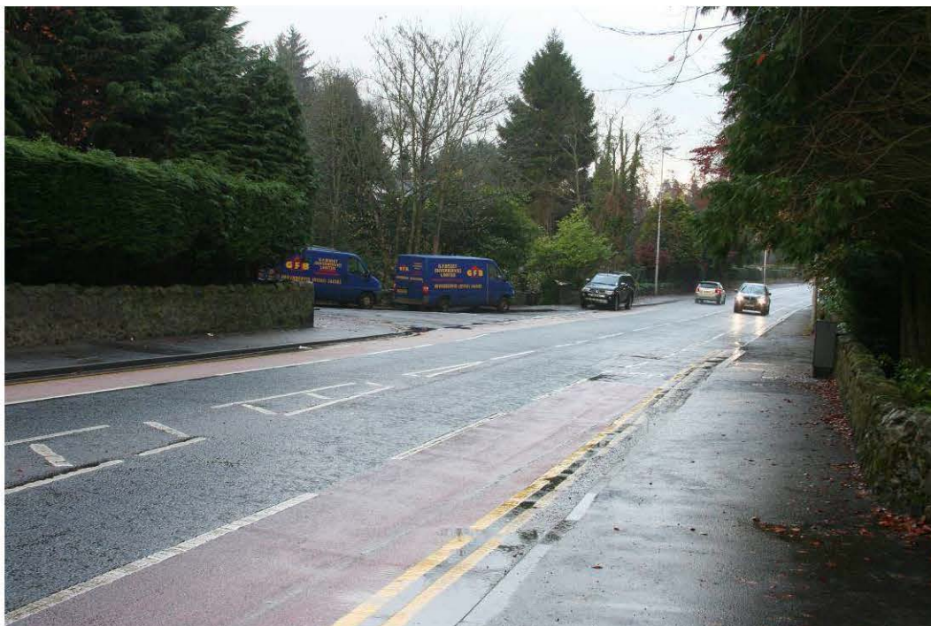
On Road Advisory Cycle Lanes on A93 North Deeside Road at Contlaw Road
