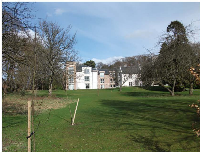
Retirement flats, Airyhall Road
