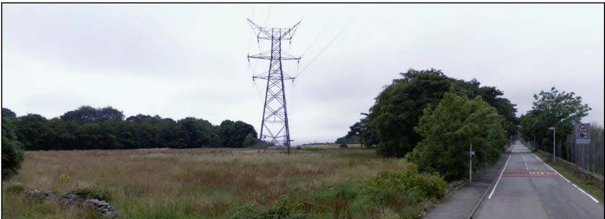
Fig 2 – the site is dominated by a line of pylons, but peripheral tree planting is of value.
