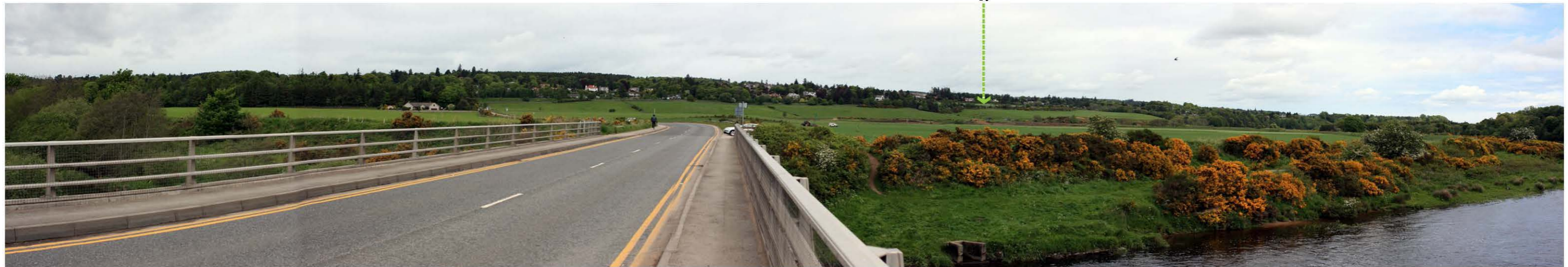
VIEWPOINT 02: B979 & RIVER DEE, LOOKING NORTH EAST TOWARDS THE SITE (GRID REF. 385846, 800389) ARROW INDICATES APPROXIMATE SITE CENTRE
