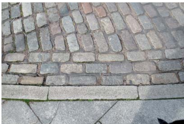
Relaid granite setts and paving, The Green
