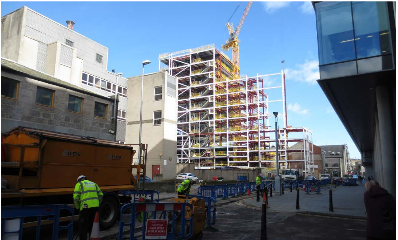
Construction of the New Capitol Office Complex
