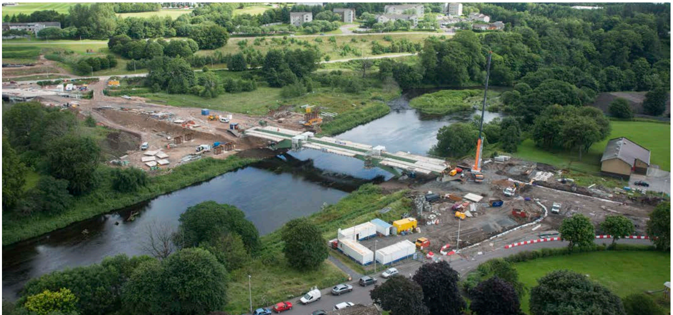
River Don, Diamond Bridge Construction
