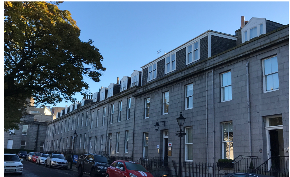
Example of a poorly designed roof extension – The modern box dormer is too large, thus it dominates the roof slope on an otherwise traditional terrace.
