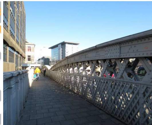
Figure 7: Guild Street Bridge
