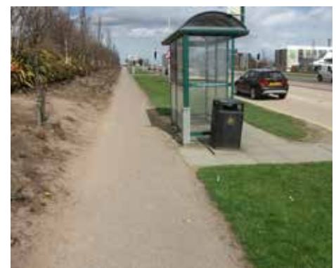
above Existing Northbound Ellon Road Bus Stop
