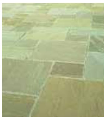
above Natural Stone Footway Surfacing
