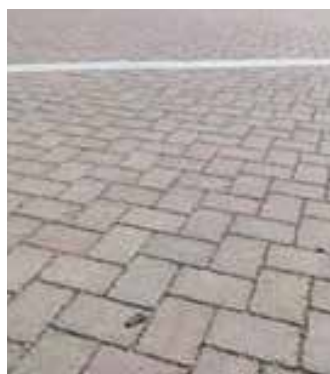
above & right Permeable Surfacing
