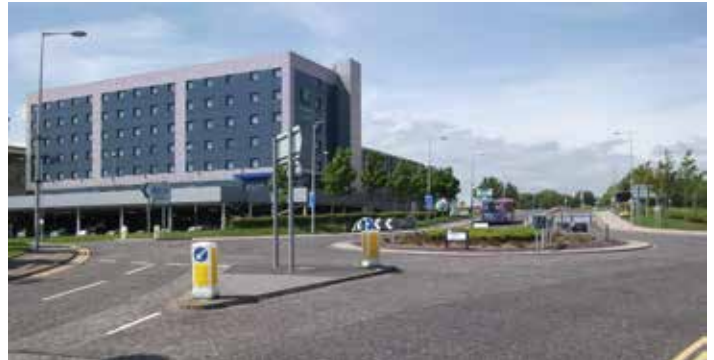
above Exhibition Avenue Access Roundabout
