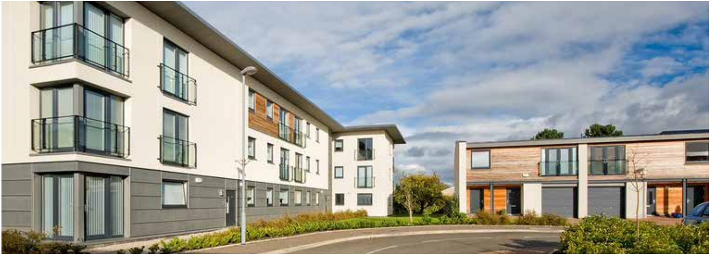
above Example image illustrating a flat roof elevation with proportional feature elements
