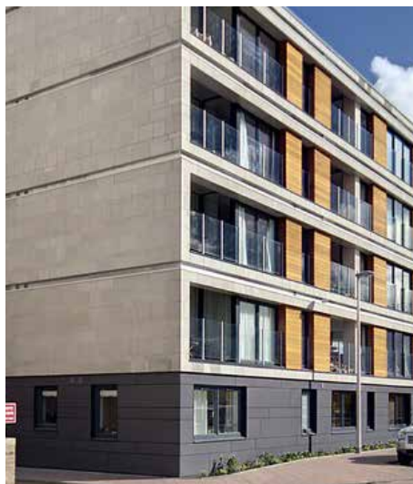
above Example image illustrating the use of Eternit cladding to base course & feature timber to balconies
