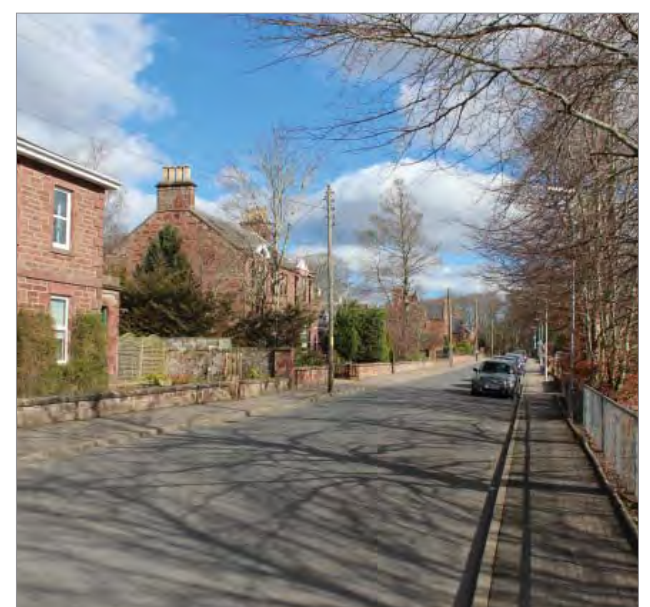
fig. 150: Detached properties overlooking street, Turriff
