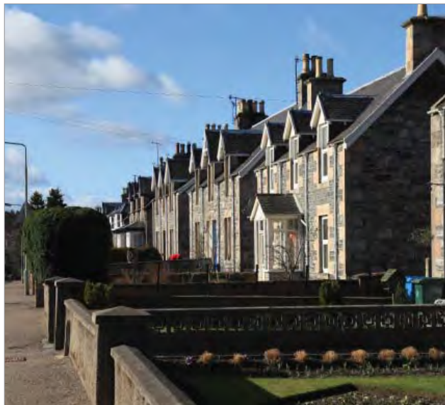
fig. 168: Residential frontage to street, Granttown on Spey
