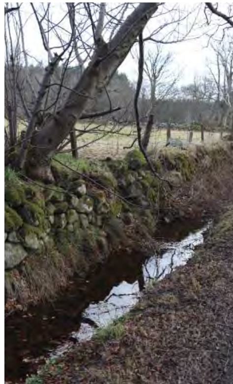
fig. 38: Existing drainage ditch adjacent Countesswells Road
