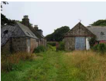
Figure 2.3 The existing farm buildings on site
