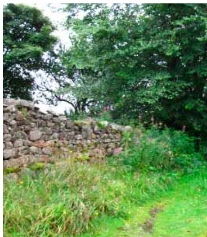
Figure 2.23 Existing stone walls on site
