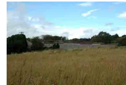
Viewpoint 17: Electricity Substation
