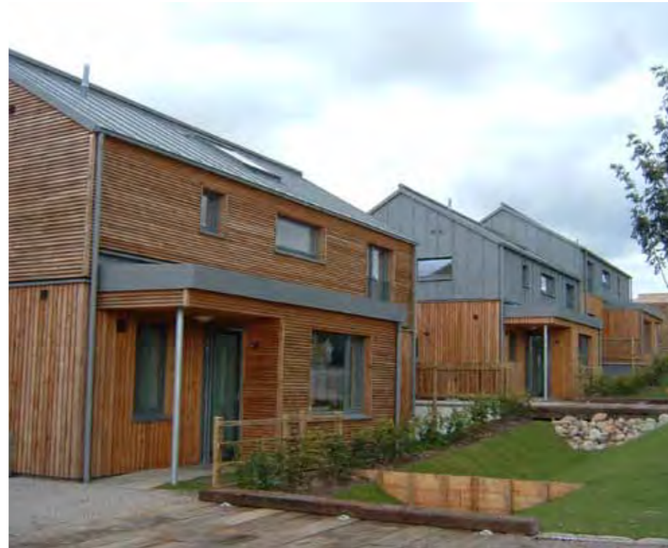
Scottish Housing Expo. Variation in timber cladding orientation and carefully considered details against window and door frames.
