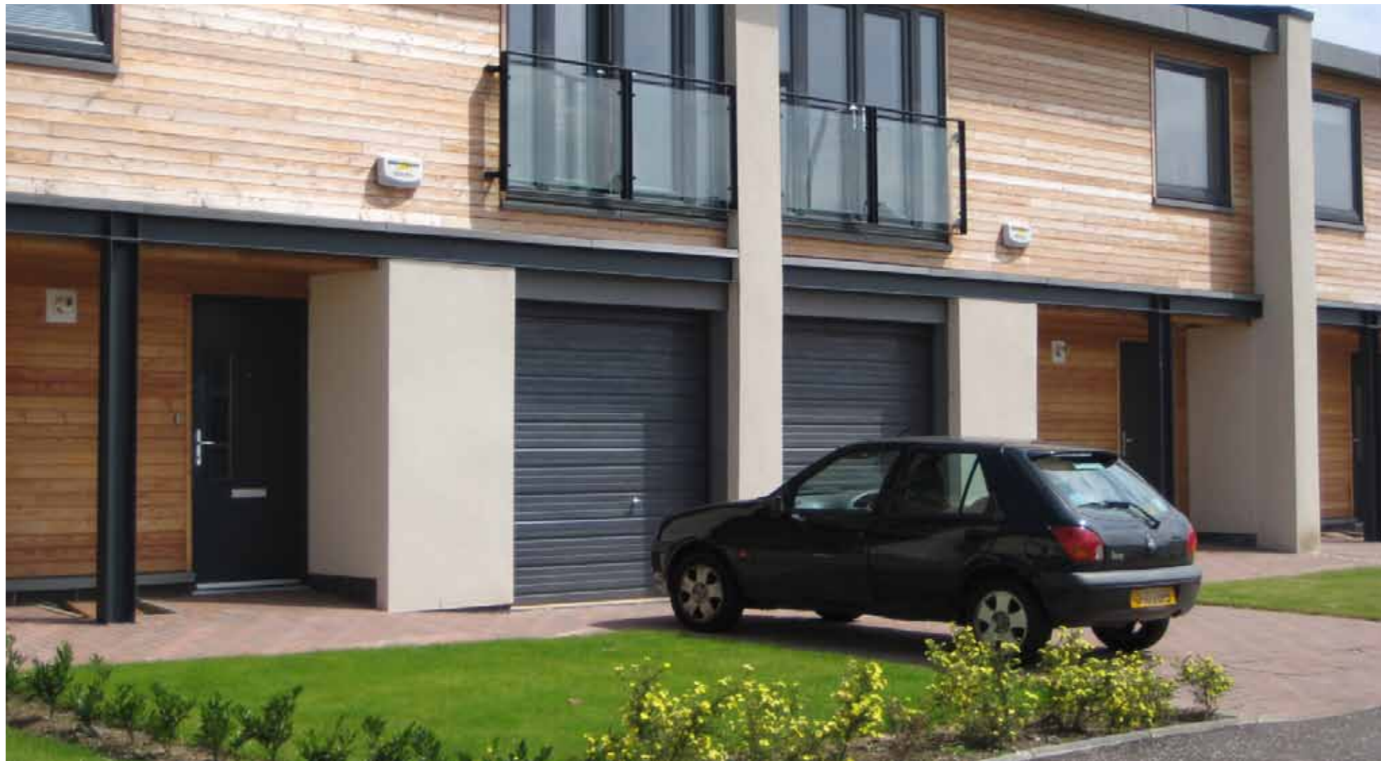
Scottish Housing Expo. Variation in timber cladding orientation and carefully considered details against window and door frames.
