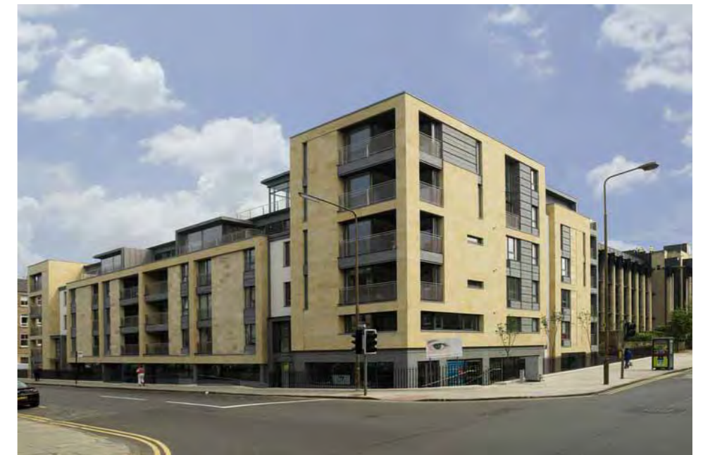
Eyre Place, Edinburgh. Eternit cladding panels at ground floor, top floor and accent areas.
