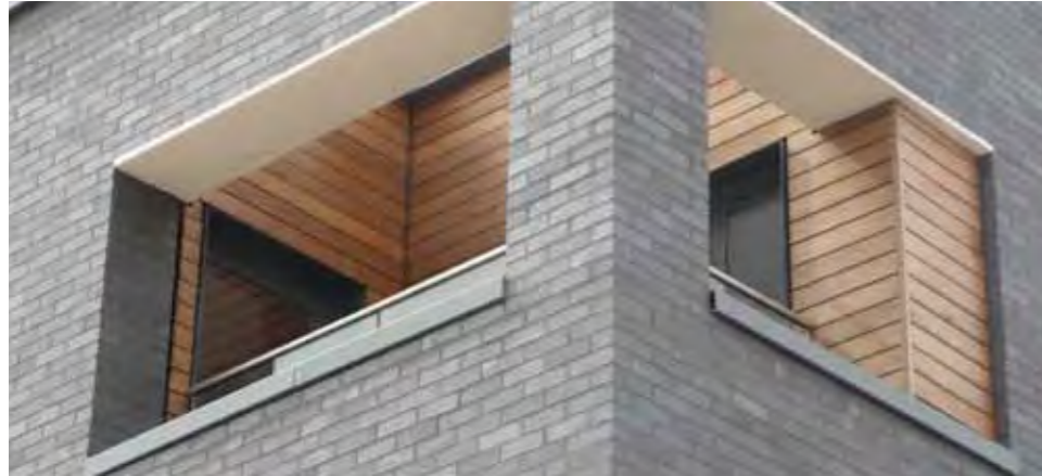
Scottish Housing Expo. Variation in timber cladding orientation and carefully considered details against window and door frames.
