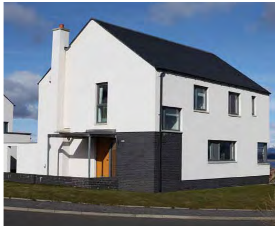
The Drum: A simple palette of white render and engineering brick unifies the development. Canopies, eaves and other projections are minimal and present relatively 'flat' modelling of elevations.
