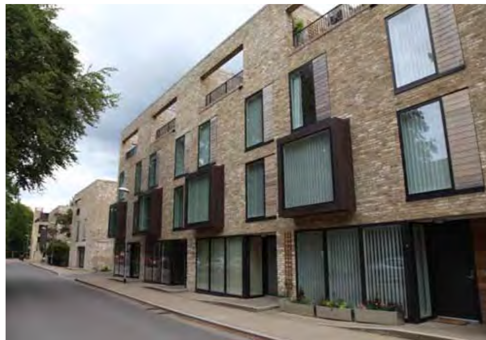
Accordia, Cambridge. Distinctive brick adopted throughout development becomes powerful element of neighbourhood identity. Thoughtful street elevations with lots of interest without being cluttered.
