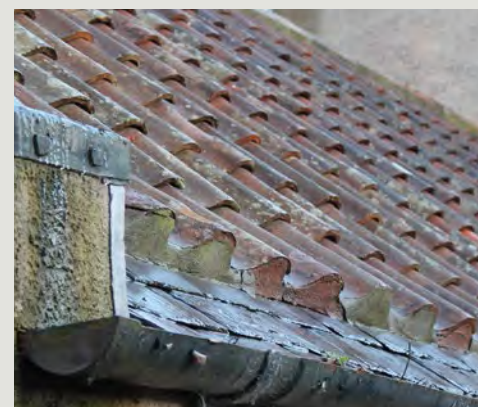
Figure 5.57: Traditional eave detail
