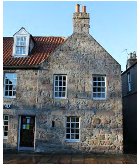
Figure 5.38: Study of Old Aberdeen mixed use building proportions informing the system used in Grandhome's single family mixed use house
