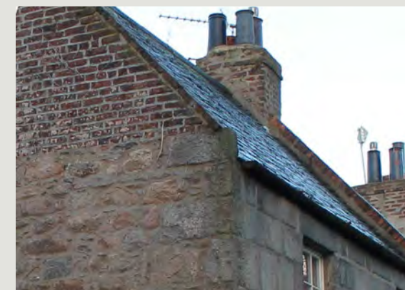
Figure 5.58: Reclaimed granite and brick gable
