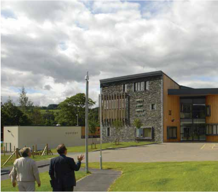
Primary school well integrated into open space with natural materials - Peebles Primary School.
