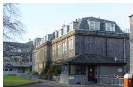
2 Boyd Orr Building
