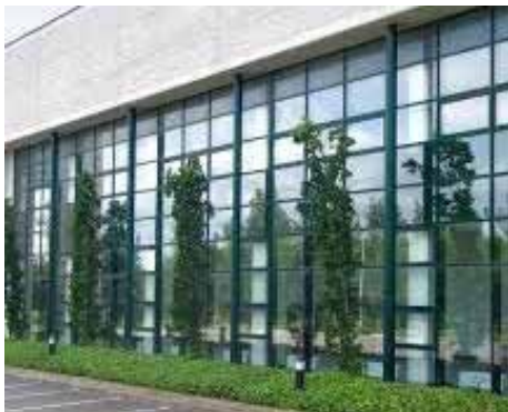
above Indicative Imagery of Capped Curtain wall system. Full height glazing to main concourse.
