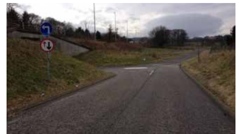
above Approach to Underpass
