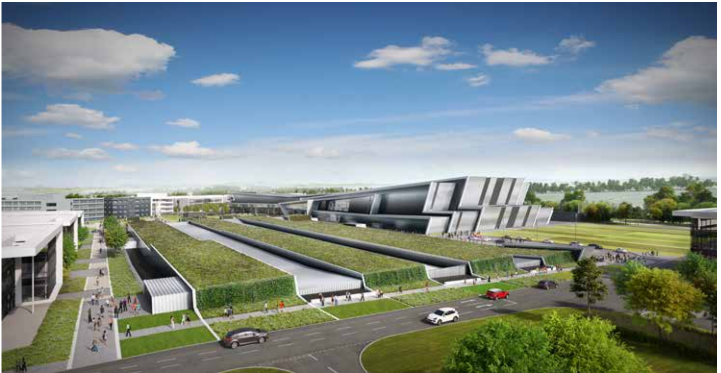
above Aerial view of Subterranean looking South-East
