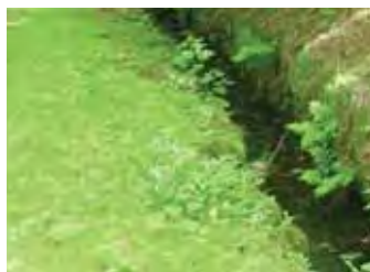
EXISTING OPEN STONE DRAINS
